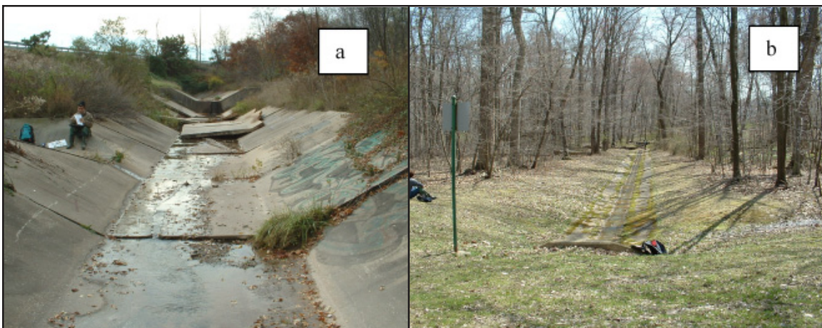
Figure 39: Restoration of Channelized Stream Segments Candidate site for structural repair (Panel A) and natural channel restoration (Panel B).
